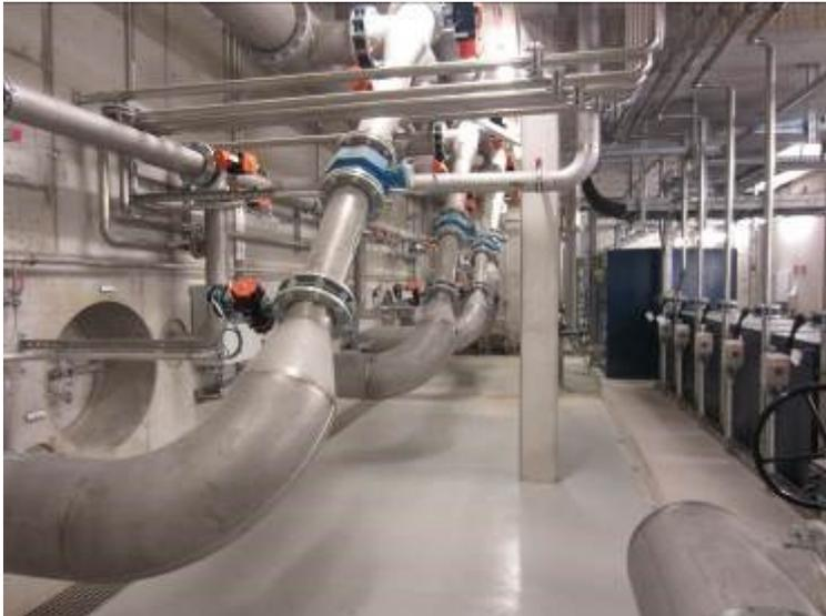
*Image 1: Inlet and Distribution to BIOFIT®.F*
