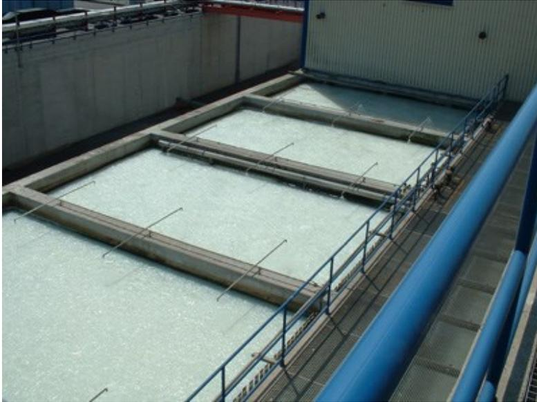
*Image 3: BIOFIT F bio filtration for additional water purification in a large paper industry project, in which Hager + Elsässer implemented their new AOP process.*
