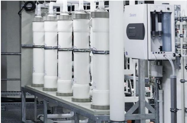
*Illustration 2: The ultrapure water membrane degassing for oxygen removal.*
