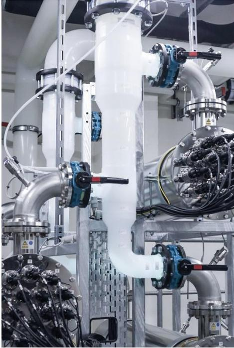
*Illustration 3: The ultrapure water UV system for TOC reduction and disinfection.*
