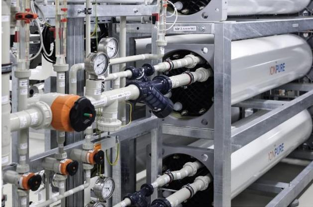
*Illustration 1: The plant produces Ultra Pure Water by combining reverse osmosis and electrodeionisation.*
